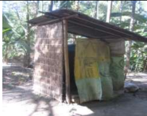
A Kucca household toilet at Behlouguri village. Such toilets are devastated after floods rendering villagers to go for open defecation
